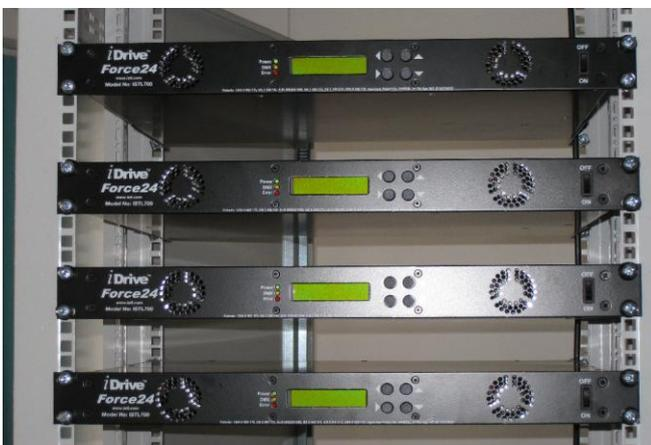
Driving electronics for luminaires
